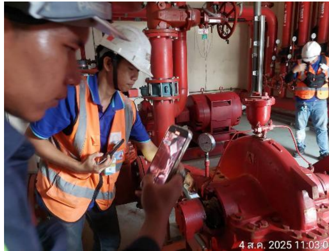
Overhaul Existing Fire Pumps & Jockey Pump
