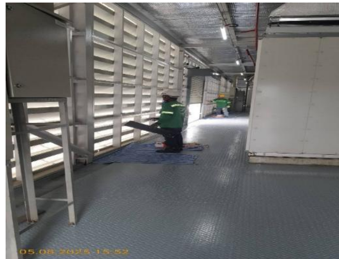
Painting Steel Structure - New AHU & OAU Building
