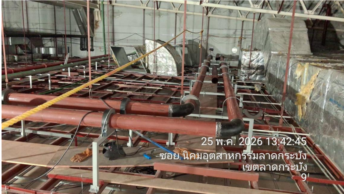
Chilled Water Piping (CHS & CHR) above Ceiling for Polym Oven
