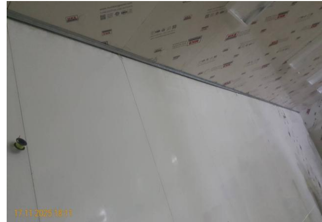
Installation of Isowall Room - Zone 5 (Hard Coat Room)
