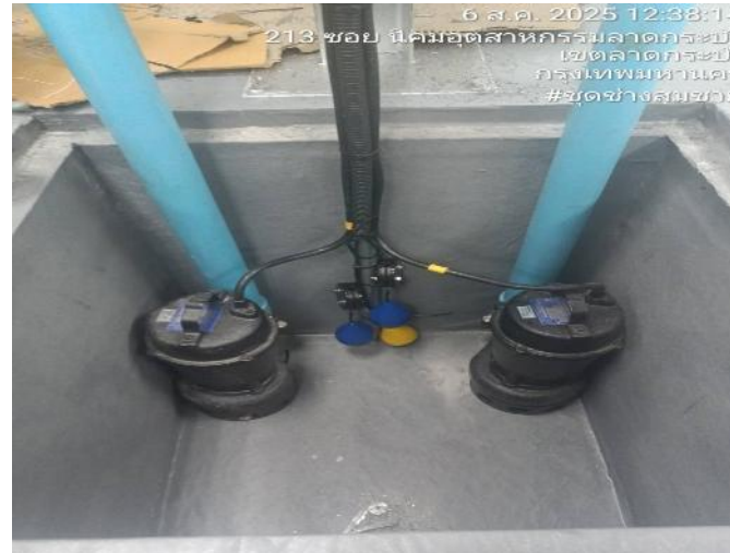
Installation of Control Pumps - Zone 2.2
