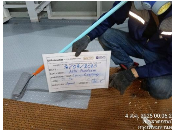
Epoxy Coating on Checker Plate Platform – New AHU & OAU Building
