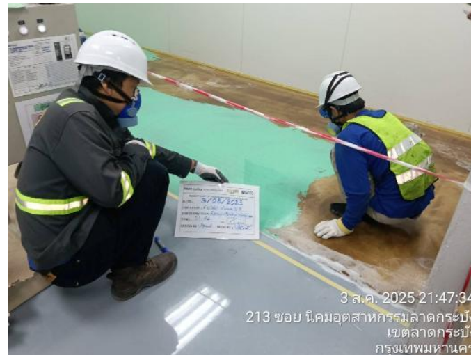
Epoxy Coating – Corridor Zone
