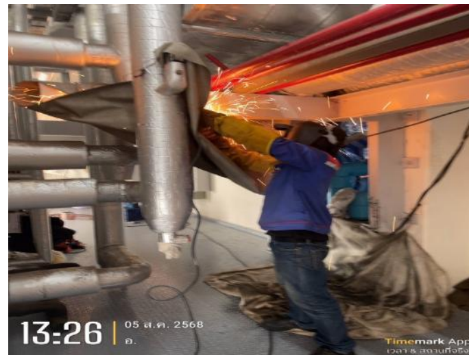
Installation of Steel Supports – New AHU & OAU Building
