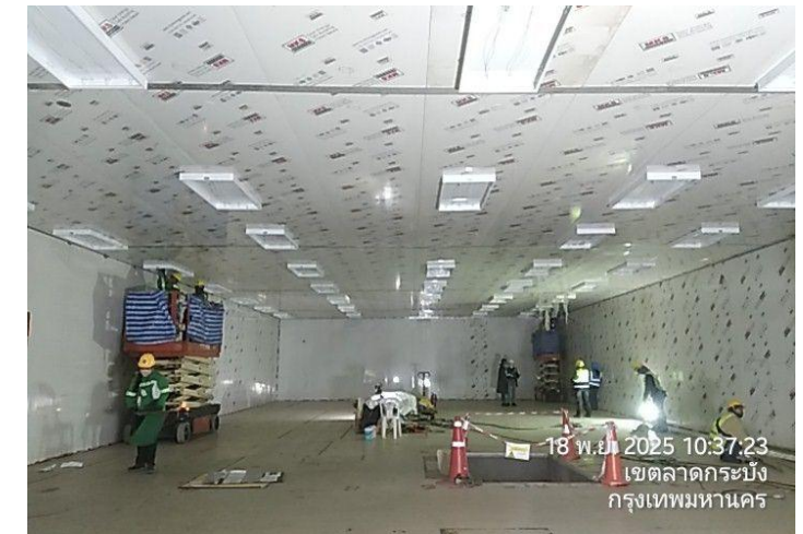
Installation of Lighting Fixture and Fire Alarm System - Zone 5 (Hard Coat Room)
