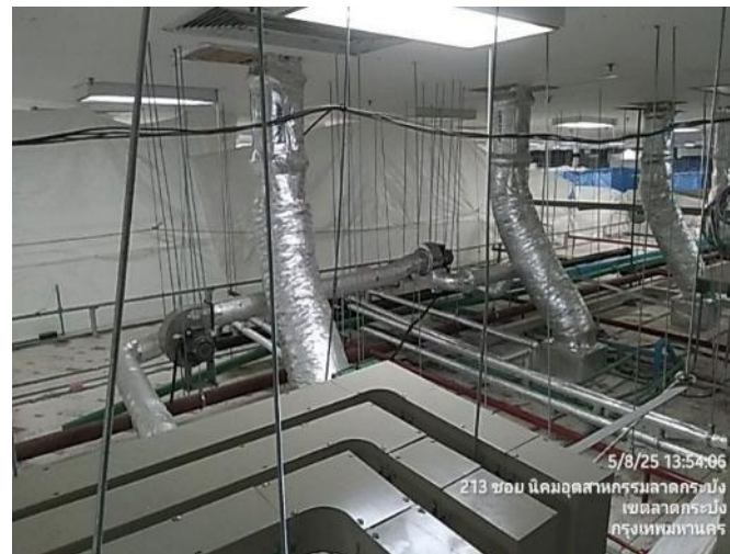
Installation of Exhaust Air Ducts - Fisa Room
