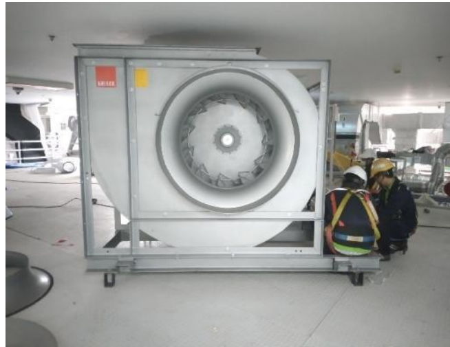
Assemble the Exhaust Fans on the Platform
