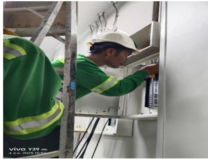
Crimping Wires into Cable Lugs for Panel Board - Assembly Room Zone
