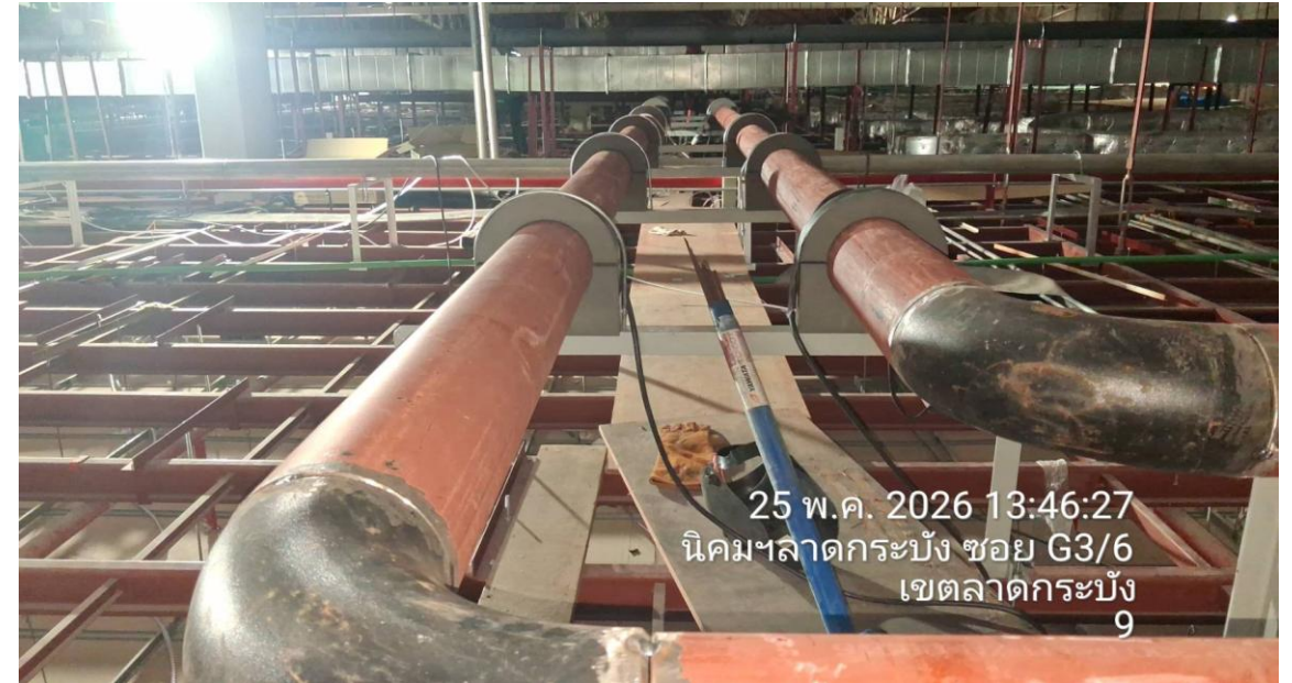
Chilled Water Piping (CHS & CHR) above Ceiling for Polym Oven
