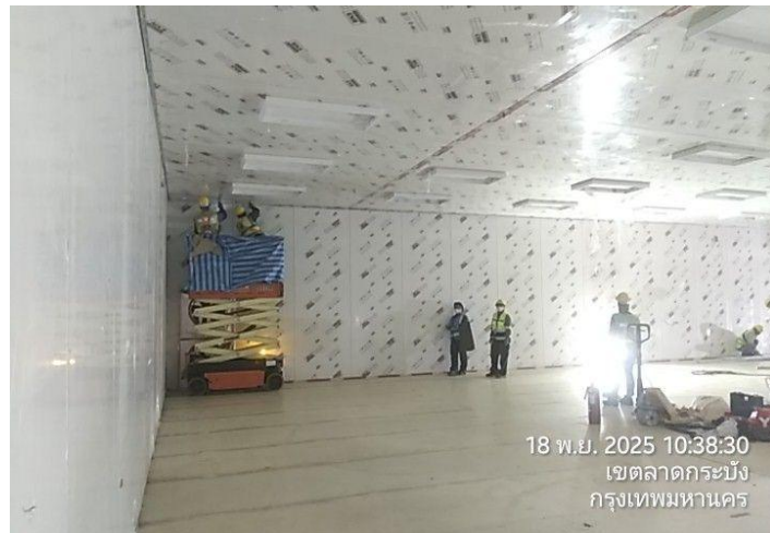
Installation of Lighting Fixture and Fire Alarm System - Zone 5 (Hard Coat Room)
