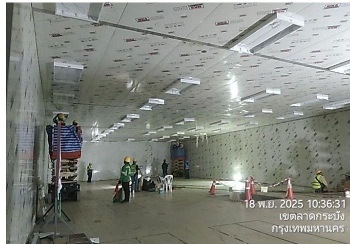
Installation of Lighting Fixture and Fire Alarm System - Zone 5 (Hard Coat Room)
