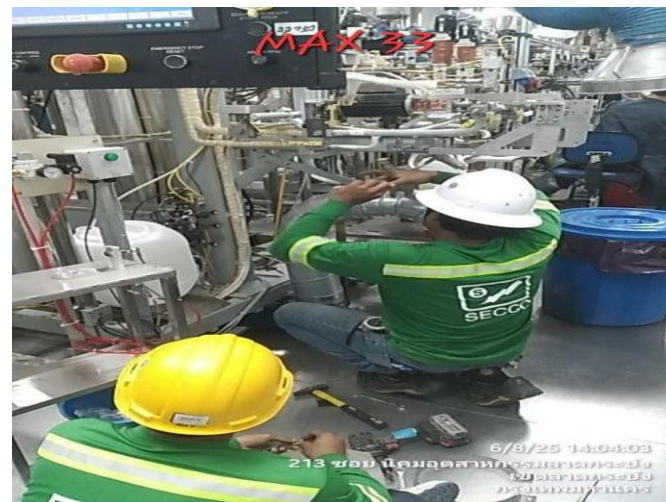
Installation of Spiral Ducts - Max 33 Machine
