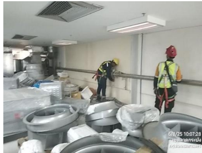
CDA Piping - Packing Room Zone
