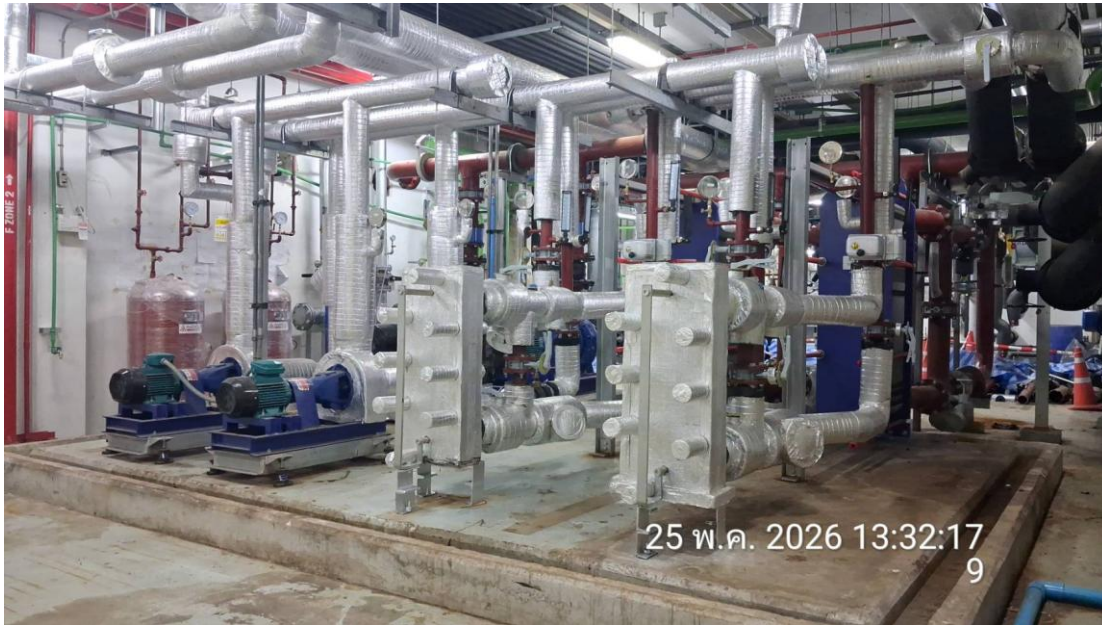
Chilled Water Pumps & Heat Exchangers
