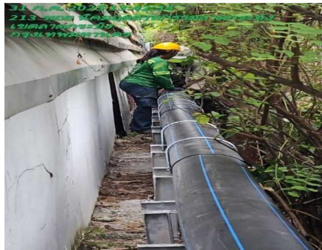
Installation of Main Drainage System – Landscape Zone
