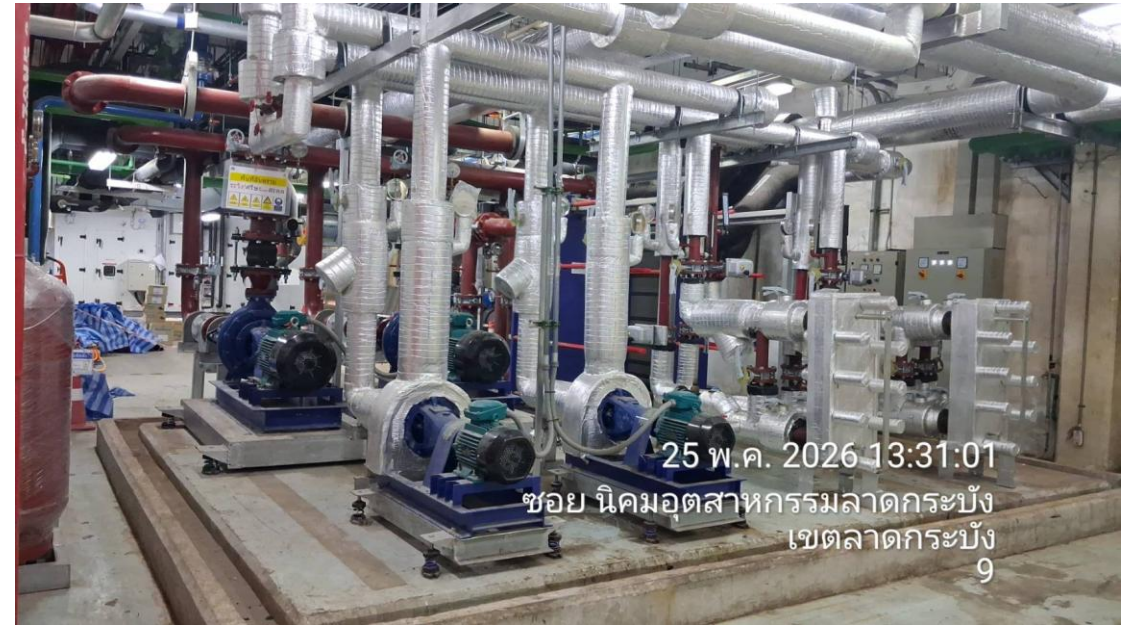
Chilled Water Pumps & Heat Exchangers
